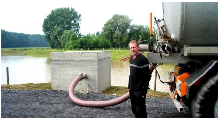
Figuur 53: Aftappunt thv bufferbekken in Vlamertinge (bron: www.focus-wtv.be )
